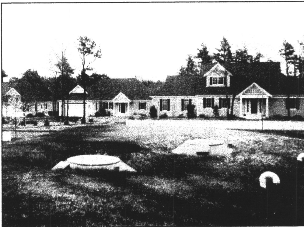
A 7,250 gpd Bioclere system serving a 24 home cluster in Cape Cod, Massachusetts. Standard effluent requirements are: 30 mg/l BOD5 and TSS, <5 mg/l Ammonia and <19 mg/l Total Nitrogen.
